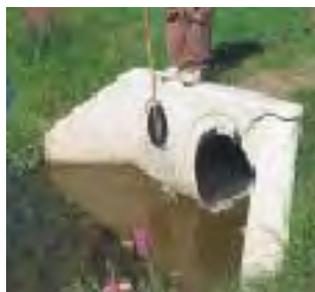
Cracked outlet pipe
