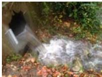
Fig. 2: Stainless Steel Compound Weir used at MC Outlet.
